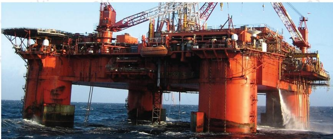
◀ Oil Drilling Ship
